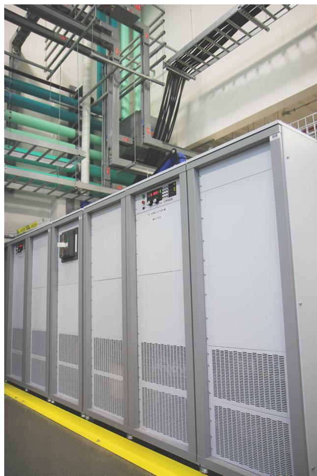
1.5 MW solar array emulator using Magna-Power MT Series power supplies at the National Renewable Energy Laboratory in Golden, Colorado USA
